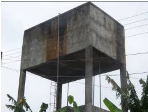
Figure 4.7 Evidence of iron in the water and broken down iron removal plant at Mampong
