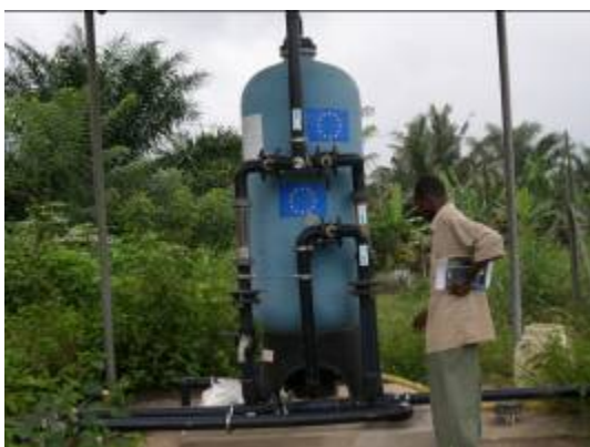
Figure 4.8 Dysfunctional iron removal plant and a High Level Tank at Assin Akropong
