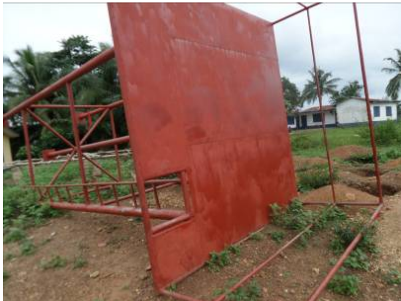
Figure 4.9 Community-funded HLT tower about to be erected at Bereku
