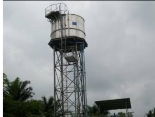
Figure 4.8 Dysfunctional iron removal plant and a High Level Tank at Assin Akropong
