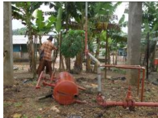
Figure 4.7 Evidence of iron in the water and broken down iron removal plant at Mampong
